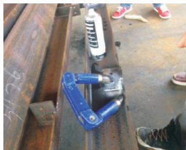
焊缝磁粉检测 Magnetic Particle Inspection at welding line
