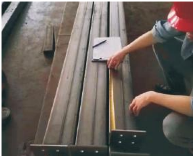
构件自检 Self Inspection
